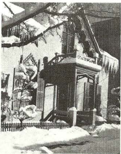
39 Front Street, Built 1857
